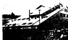
Successfully Operating Large Tungsten Mill Engineered and Built by Denver Equipment Company
