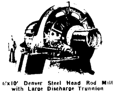
6'x10' Denver Steel Head Rod Mill with Large Discharge Trunnion
