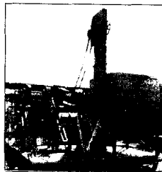
Denver Belt Bucket Elevator Installed in Denver Mill
