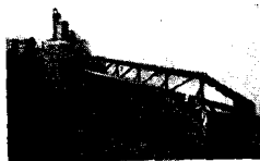
Truss Type Superstructure for Denver Spiral Rake Thickener—Note Duplex Denver Adjustable Stroke Diaphragm Pump Mounted on Superstructure in Background
