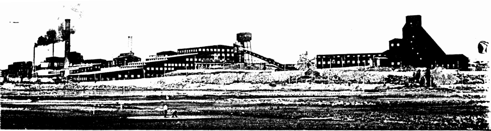
Mill of the Hudson Bay Mining and Smelting Co. at Flin Flon, Manitoba, where Merrill-Crowe Precipitation and Mills-Crowe Cyanide Recovery are utilized in the cyanidation of a low grade pyritic flotation tailing.
